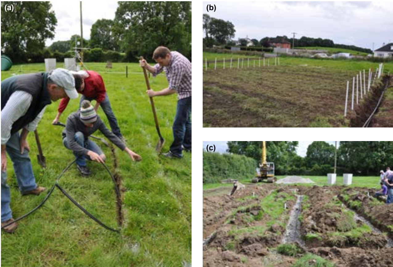
Figure 2.15. (a) Installation of DD tubing, (b) final DD installation at Site B and (c) installation of LPP at Site A.
